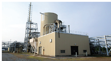
Pine Bluff Integrated Binary Production Facility
