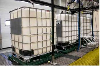
After chemical warfare materiel is neutralized, liquid waste is drained from the vessel of RCMD's Explosive Destruction System (EDS) to 55-gallon waste drums, which make up the EDS waste transfer subsystem.
