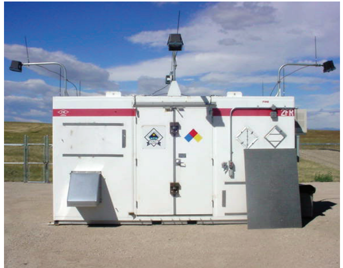
The interim holding facility provides safe storage for recovered chemical warfare materiel.
