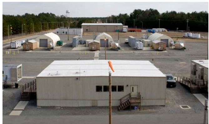
Three separate Environmental Enclosures house the transportable Explosive Destruction System units. The facility is known collectively as the Pine Bluff Explosive Destruction System, or PBEDS.
